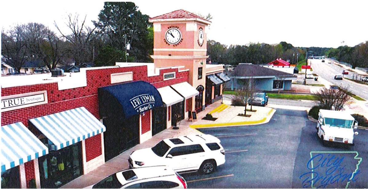
"Old Town" Shopping Center - Reynolds Road
