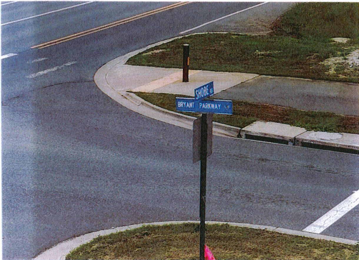
2023 Improvements - Starting point of Bryant Parkway Phase II
