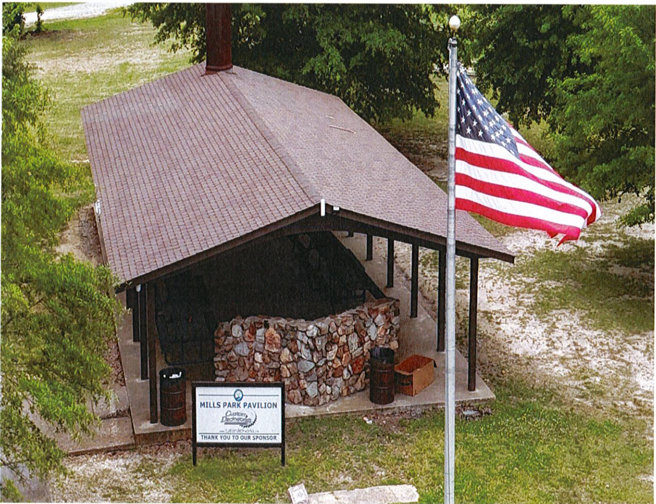
2023 Improvements - Mills Park Pavilion
