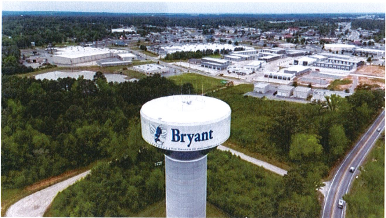
Bryant Water Tower, Hwy 5, South View
