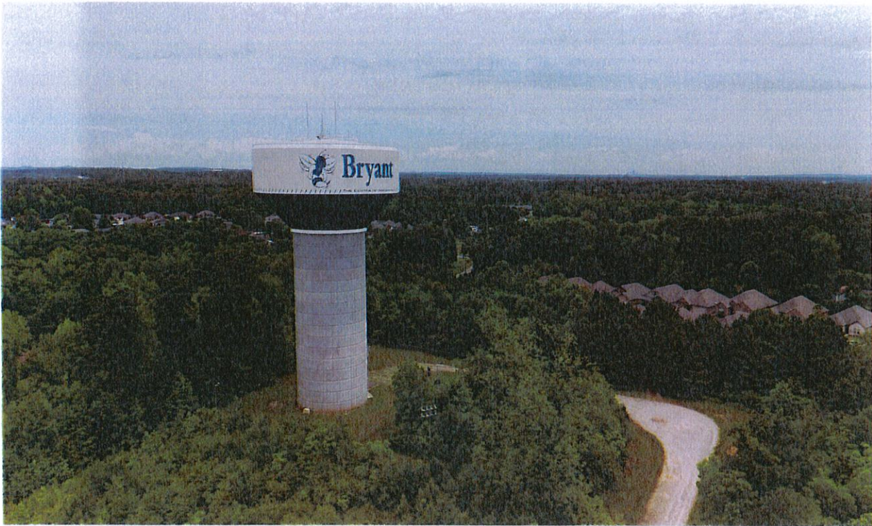
Water Tower, Hwy 5, North View
