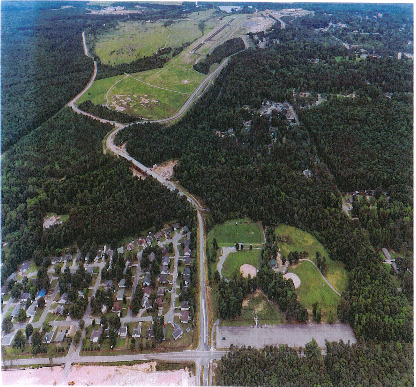
2023 Work in Progress - Bryant Parkway Phase II
