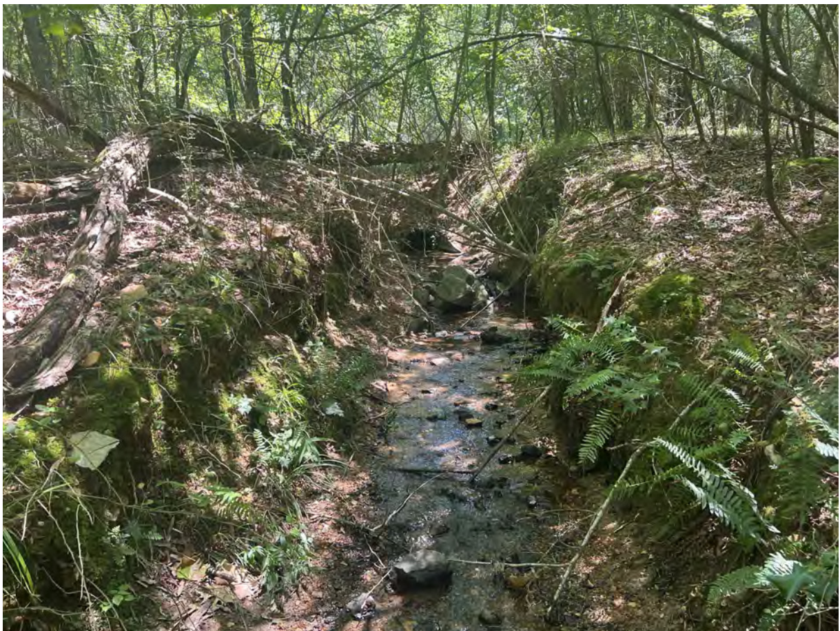
PHOTOGRAPH 20 — VIEW OF INTERMITTENT STREAM A CULVERT LEAVING POND A.
