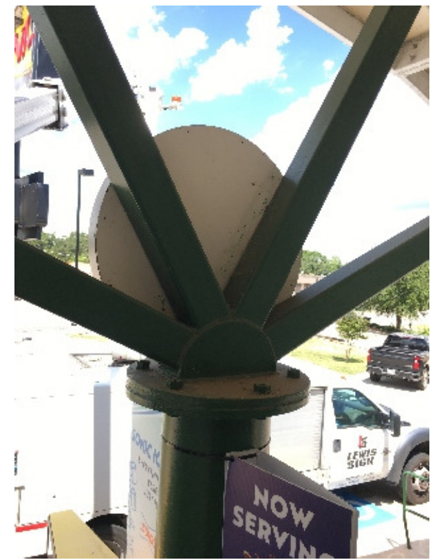
EXISTING SIGN- TO BE REMOVED/BACK VIEW OF BRACING
