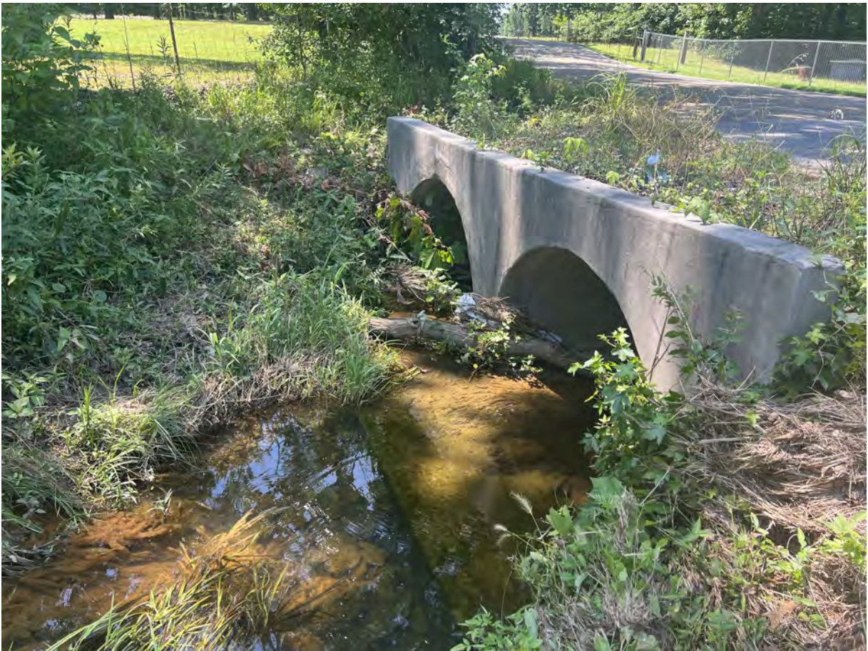
PHOTOGRAPH 24 — VIEW OF INTERMITTENT STREAM A LEAVING SITE.
