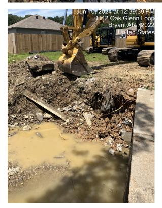
On June 10th, PW started construction on the Oak Glenn/Crossing Loop Box Culvert removal. The culvert install was required when the subdivisions were constructed for emergency personnel access. This area has been identified as a bottleneck for the creek at times of high flow due to varying storm events.
