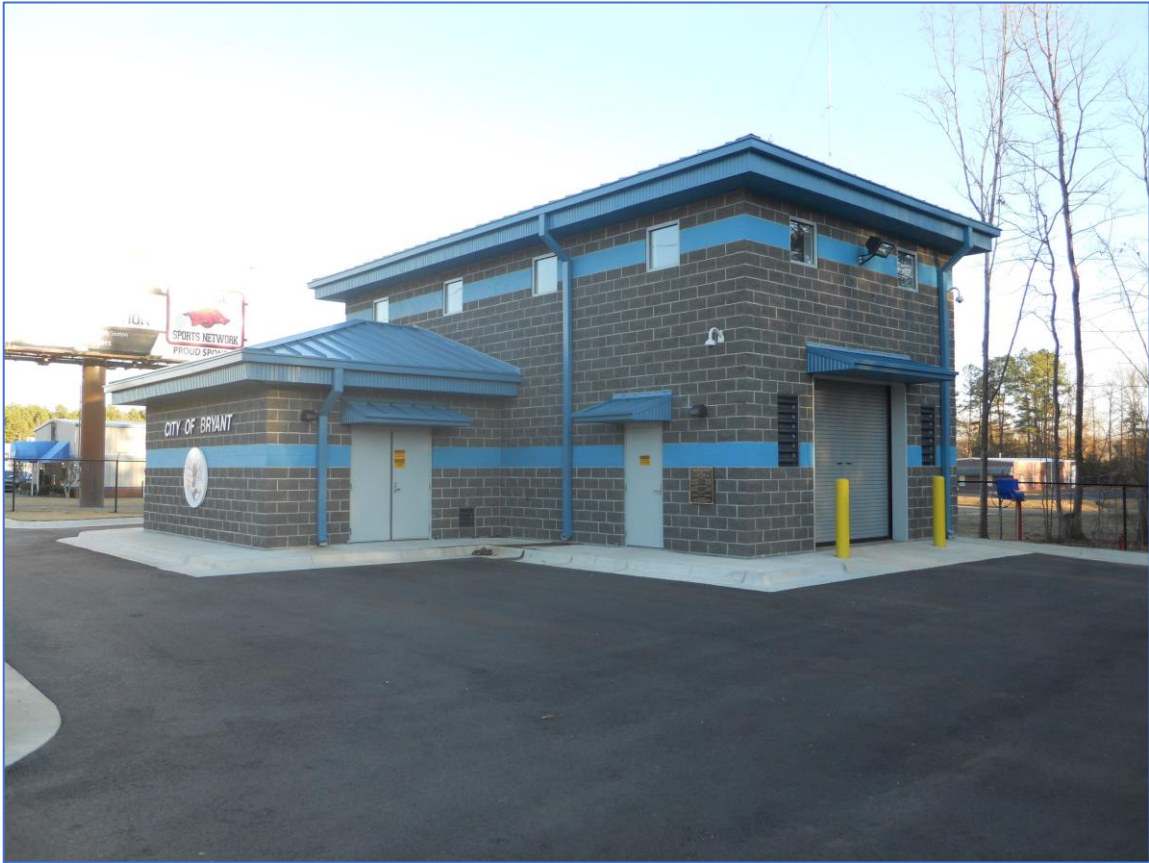
Figure III-3: Booster Pump Station
