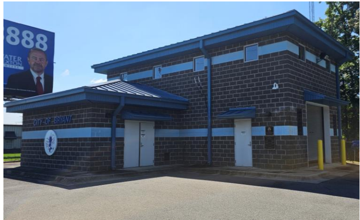
Figure II-4: Bryant Booster Pump Station
