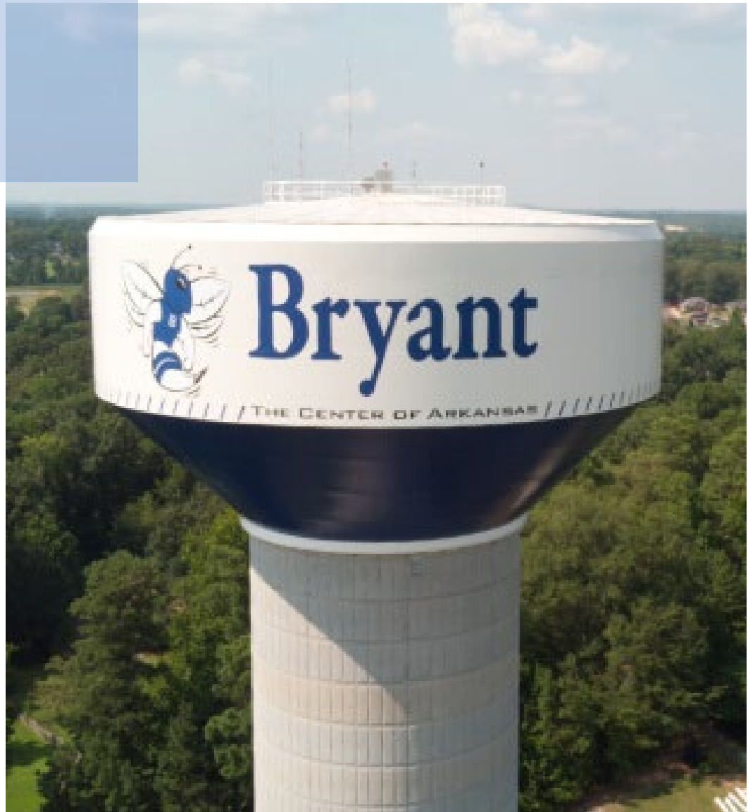
Bryant Water Tower, Hwy 5
