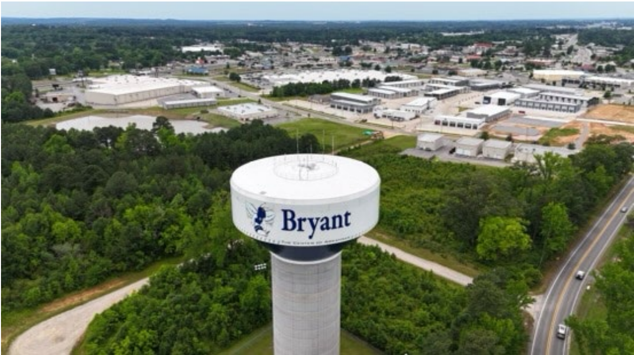
Bryant Water Tower, Hwy 5, South View
