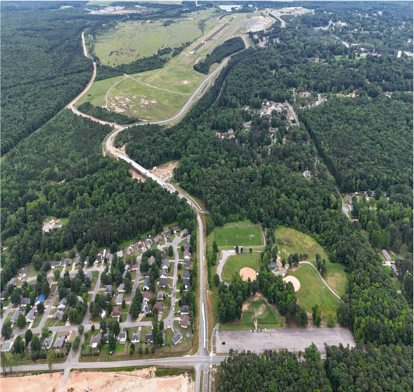
2023 Work in Progress - Bryant Parkway Phase II
