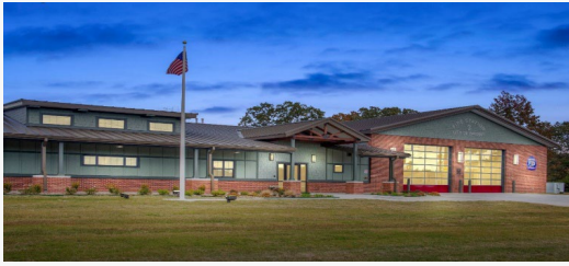
Station 3 located at 2620 Northlake Road covers Fire District 3 and the Springhill Fire Protection Area
