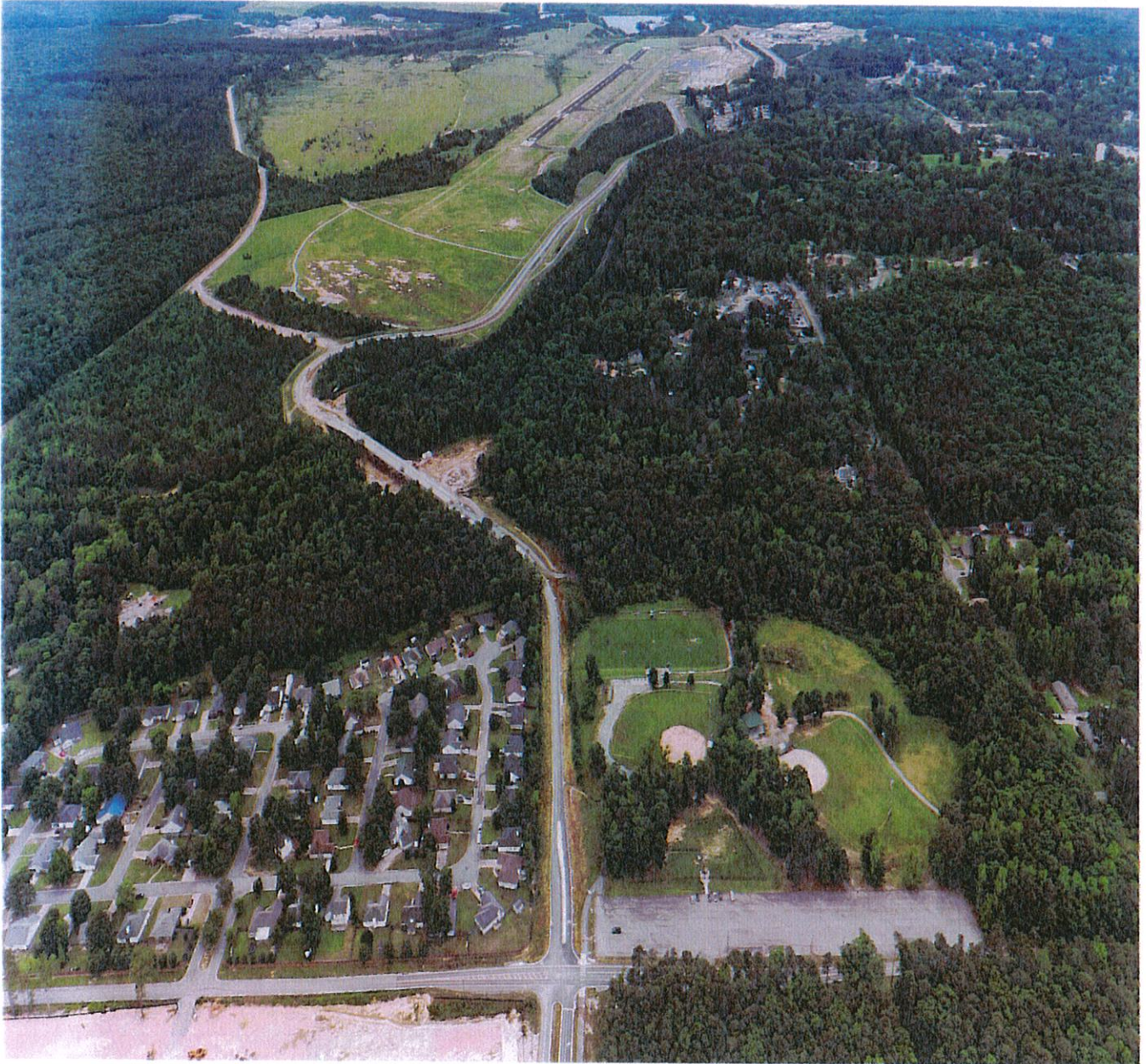
2023 Work in Progress - Bryant Parkway Phase II
