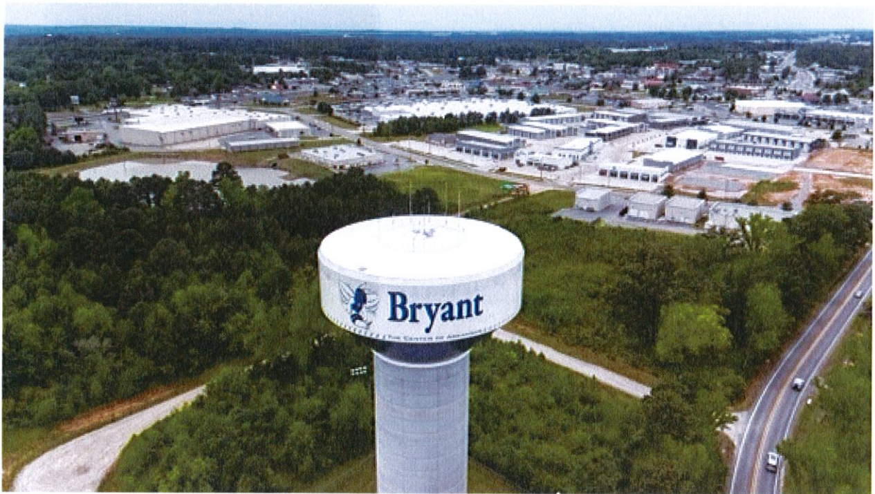
Bryant Water Tower, Hwy 5, South View
