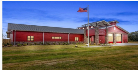
Station 2 located at 1601 South Reynolds Road covers Fire District 2
