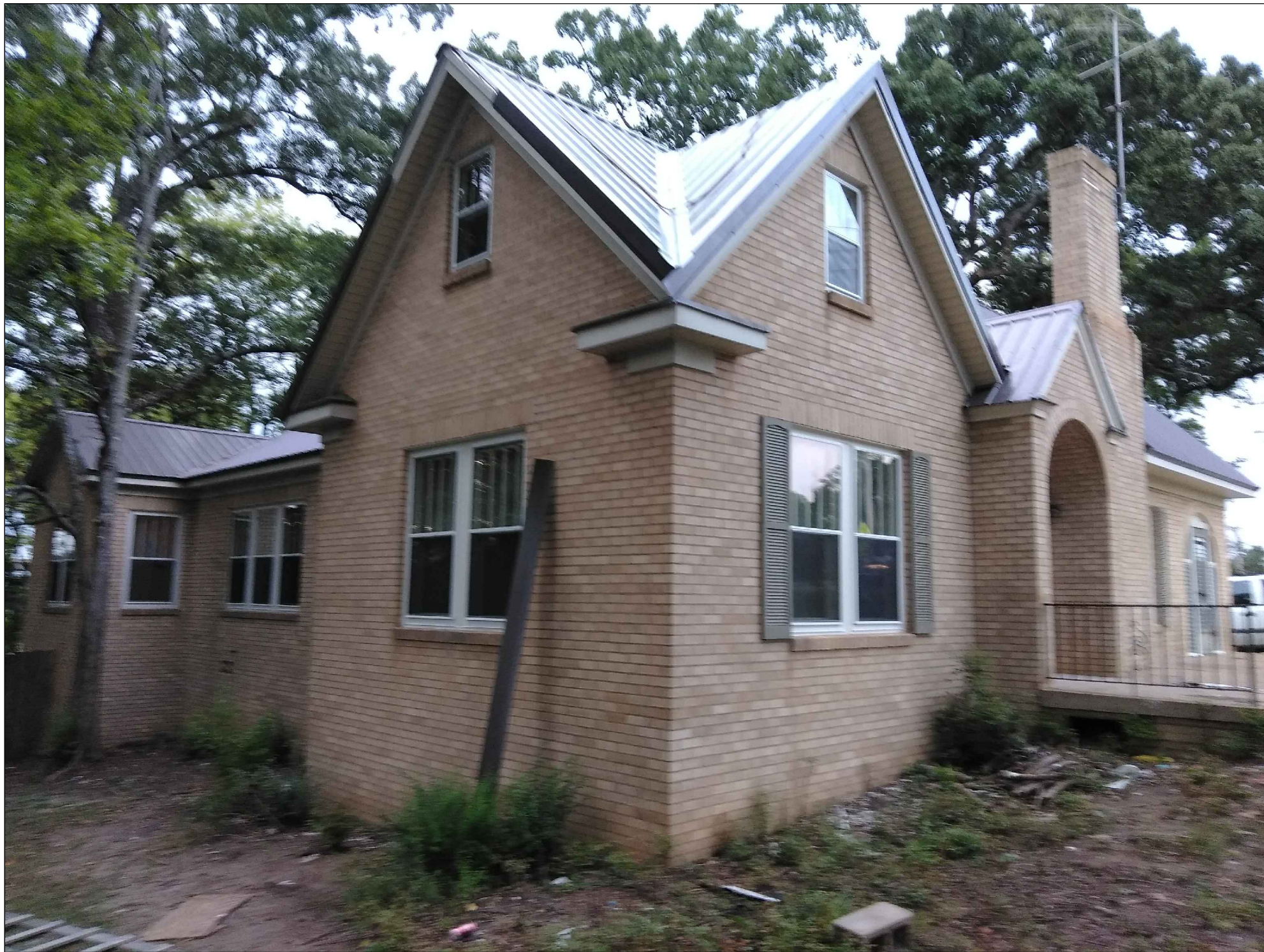
STREET VIEW OF EXISTING SOUTHEAST CORNER OF BUILDING
