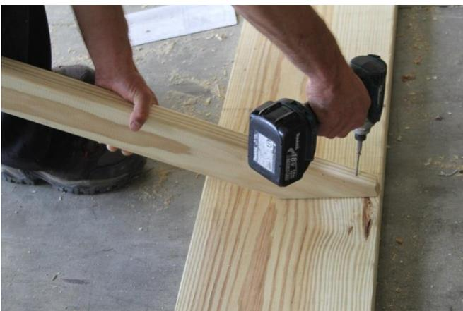
11. Next, attach the bottom of this rafter to the top plate as done with the other rafters, using 3 ½" screws one through the top and one through the side. Follow this process for the other side as well.
