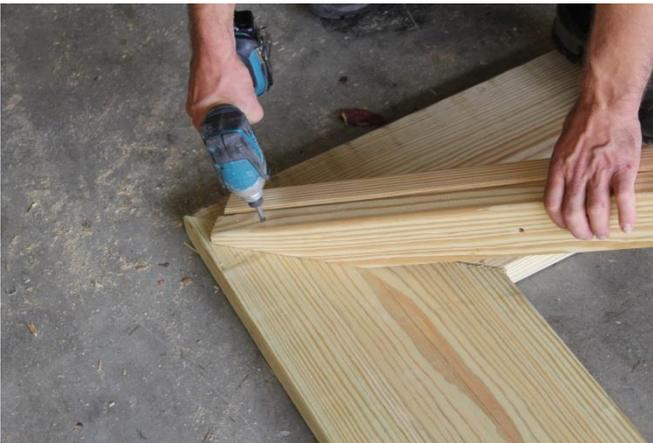
13. Next, set the bottom of these two boards centered on the top plate and up against the fascia. Once in place, screw these rafters into the top plate with 3 1/2" screws, one in the top of each rafter and one through the side. Follow this process for all four corners until all the bottoms of the corner rafters are attached.
