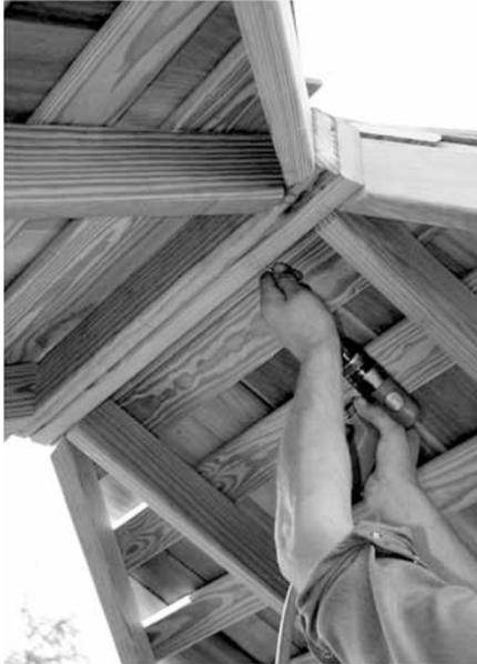
24. Once you have both sections set into place you will need to raise both panels so they mate at the ridge. Make sure that you have a helper tending to the props so that they do not get dislodged during this process. With the roof panels aligned and flush with each other, you will want to secure them together with 2 ½" screws. At this time please do not attach the rafter to the top plate.
