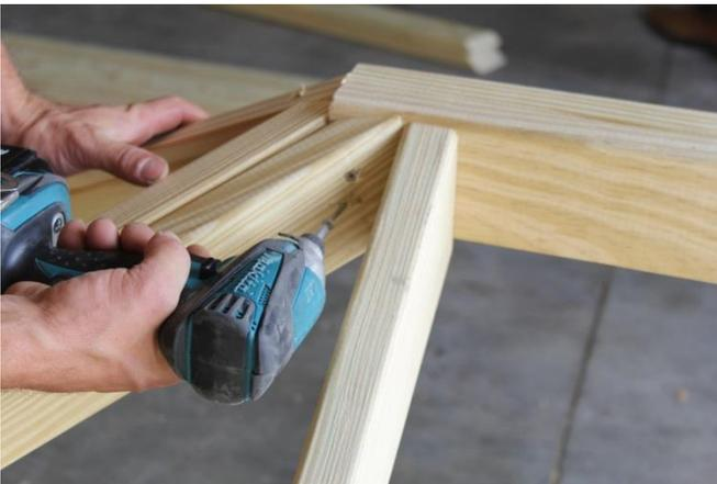
14. Then take the tops of the corner rafter and set them against the ridge board as shown. Once in place, screw them into the top plate with 2 1/2" screws two from each rafter into the top plate. Do this until all the corner rafters are installed.
