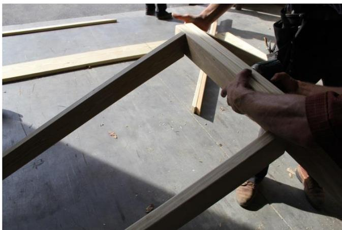
7. When everything is flush, connect the two ridge boards together using 2 ½" screws. Place a screw about every 10-12 inches, making sure to do this on both sides of the ridge boards.
