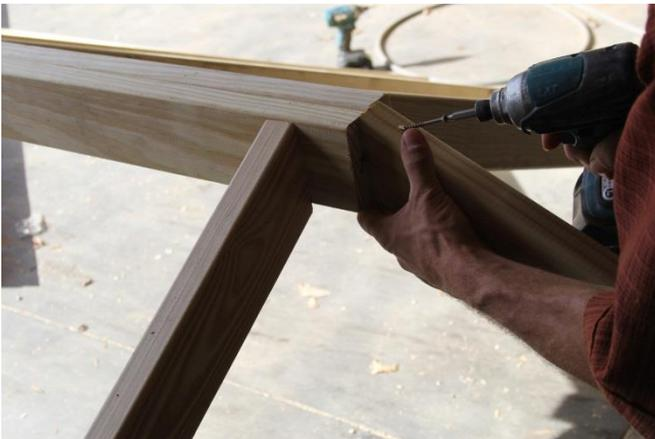
10. Now, take this rafter and place it on the center of the two ridge board ends, making sure that it is flush with the top. Then connect the rafter to the ridge boards with a 2 ½" screw from the top and one from each side.
