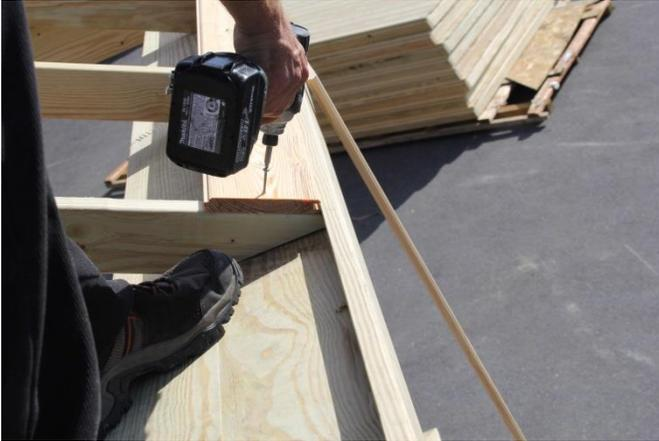
20. When the first is board cut and set into place, screw it into each rafter with a 2 ½" screw in the center of the T&G decking board. Follow this process on all sides of the roof until it is fully covered in decking. Once this is done you are ready to install the shingles.
