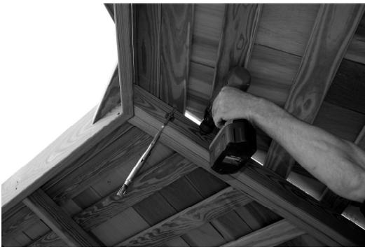
Tip: You can use several aides in aligning the rafters. A clamp is very handy in keeping the rafters aligned until they are secured to each other.
