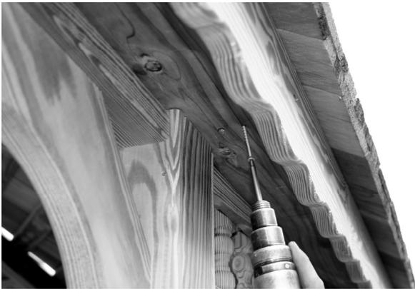
26. To fully secure the rafters to the top plate you will need to drive a 3 ½" white headed screw from the bottom of the top plate up into the rafters. You will want to insert the screws 1" from the outside edge of the top plate. Do this around the entire Gazebo at every rafter. The roof is now complete and is ready to have the ridge capping installed.
