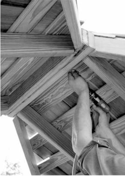
36. Once you have both sections set into place, you will need to raise both panels so they mate at the ridge. Make sure that you have a helper tending to the props so that they do not get dislodged during this process. With the roof panels aligned and flush with each other, you will want to secure them together with 2 ½" screws. At this time please do not attach the rafter to the top plate.
