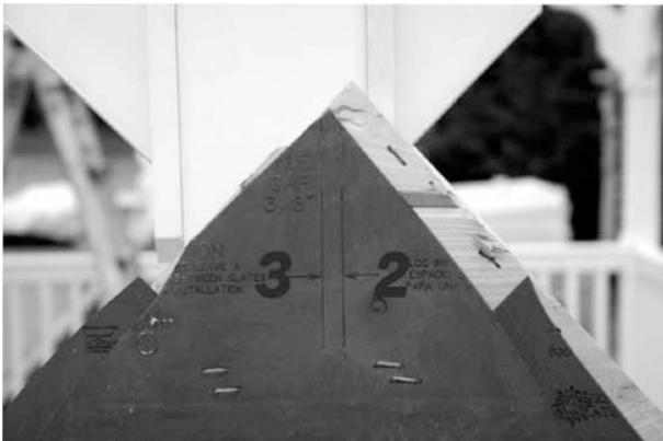
20. You will notice that all of the roofing sections are labeled and have two numbers on them. You will want to find the sections with the same numbers and match them together. Also you will notice that some of the roofing sections come to a point at the top and the others are flat. The sections with the flat ends are the longer sides of the front and back. They go together first.
