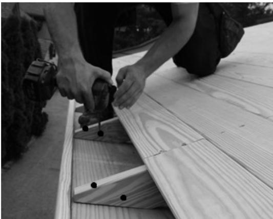
40. Once all of the rafters are attached to the top plate, you can now re-attach the roofing boards that you previously removed. And now you are ready to install shingles on the roof.
