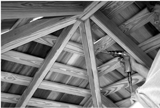
37. Next raise an adjoining panel into position, (a prop is handy in aligning the end panel with the main panel.) Keeping the end panel/rafter flush with the adjacent panel/rafter, secure them every 24" using 2 ½" screws. Do this for all roofing panels.
