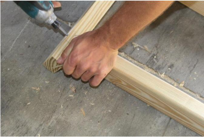
4. Now, take the ridge board and place it on top of the angled cuts that are flush on the ground with rafters as shown, making sure to have a rafter against the X marked on the ridge board. Next you will connect the ridge board to the rafters with 3 ½" screws, two per rafter.
