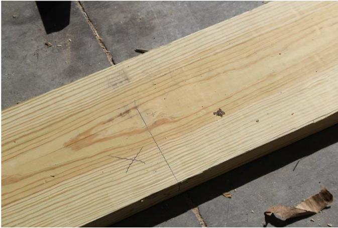
5. When this is done for both sides of the center sections, look at the top plate board and see another set of X's with lines beside them. This will be your guide as to where the other ends of the rafters that were just connected to the ridge board, will then be connected to the top plate.
