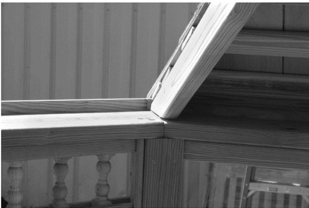
34. Align the rafters with the edge of the top plate, resting against the fascia.
