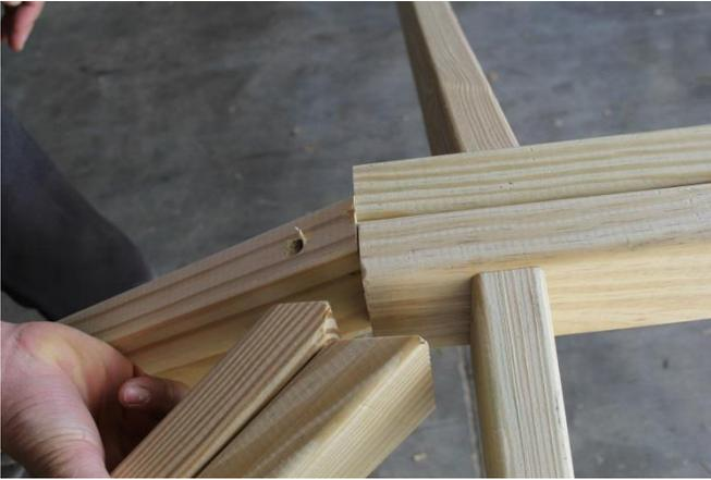
12. Now, install the corner rafters, these are usually a set of two boards that are attached together. One will have a pointed cut on the top and the other will have an angled cut. (See picture to the left)
