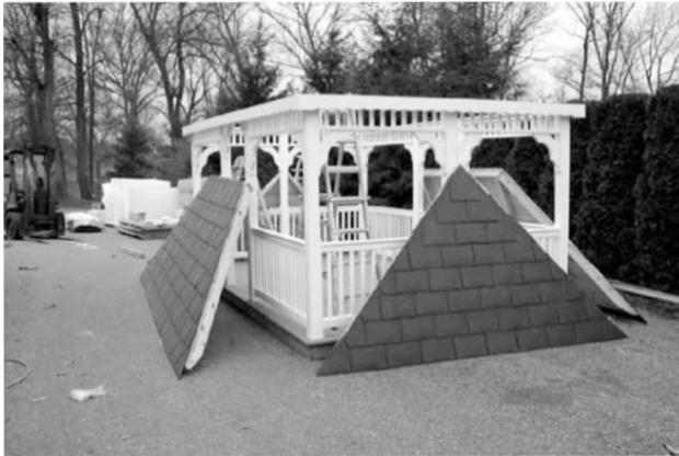
19. Place the roofing sections around the building. (NOTE: The picture shows rubber roofing already on the Gazebo. If you have an asphalt roof, the roofing sections will only be tongue and groove and the shingles will not be on.) NOTE: If you have Cedar Shakes or Rubber Shingles follow steps 20 to 26. If you have Asphalt Shingles or Metal Roofing follow steps 27 to 37.
