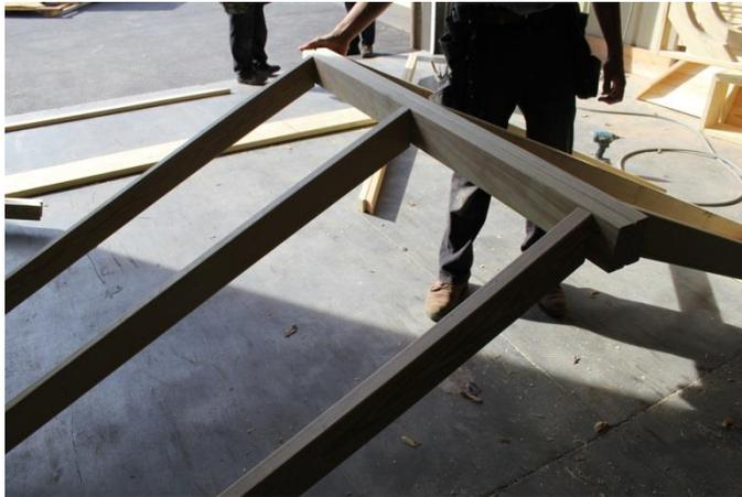
6. Next, take the ridge board and center rafter sections and rest the ridge boards of the two sections together. Once they are resting against each other, make them flush on the ends and also on their tops. (please use the picture at left as a reference)
