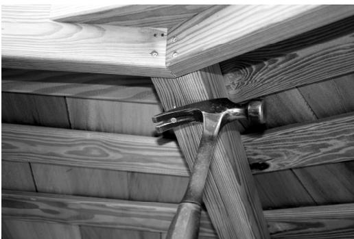
Tip: Also to pull a panel into position for alignment you can drive a screw into the higher panel/rafter and using the claw on a hammer pull it down into position.
