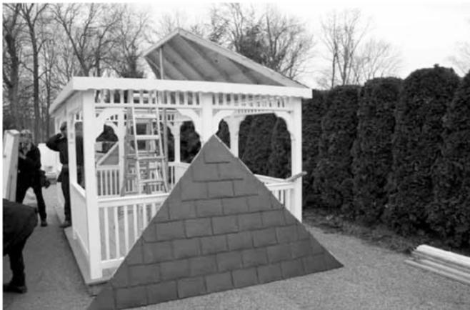
23. After you have the first section in place you can use a prop board to hold it into place while you get the second long sided roofing section set into place. If you use a prop make sure that you place it toward the inside of the roof panel, so you do not have the chance of it see-sawing.
