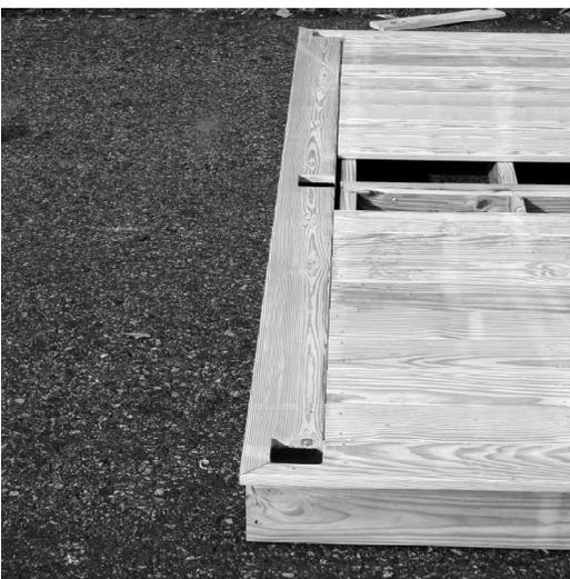
6. Now you will want to set the missing top decking boards into place, you will notice that they also have letters for proper placement. You will want to screw these decking boards into place with 2  $\frac{1}{2}$ " screws. (If you have composite decking you will use the screws that are the same color as the deck)
