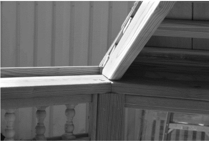
22. Align the rafters with the edge of the top plate, resting against the fascia. **NOTE:** Make sure the bottom cut is setting flat on the top plate.
