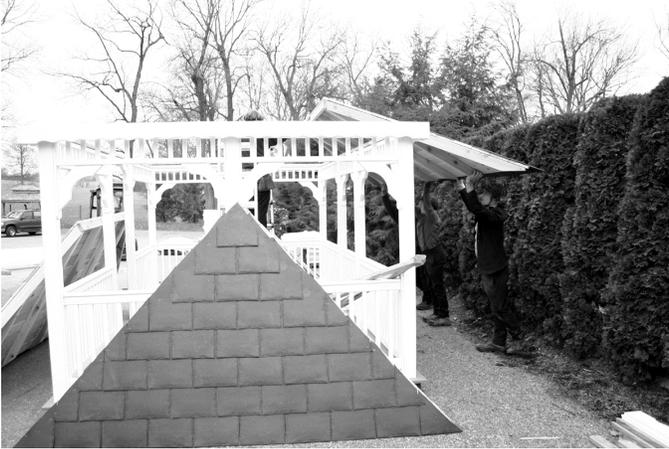
21. First raise a long side panel up onto the top plate. Slide this section up until the rafters in the roof drop into the top plate while resting against the inside of the fascia.
