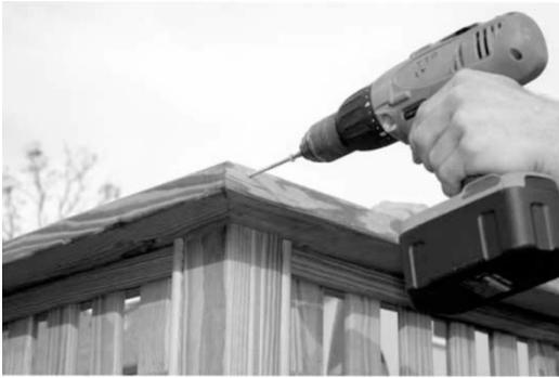
15. Position the adjoining top plate for installation and screw it from the corner to the other top plate. Follow these steps until all the top plates are in place. Make sure all corners fit tight and are spaced evenly over posts. \*You may need to un-screw the first board to get the tight fit. Then you will want to fully secure the top plates from the top by driving a screw every 16" the entire length of the top plates with 2 ½"
