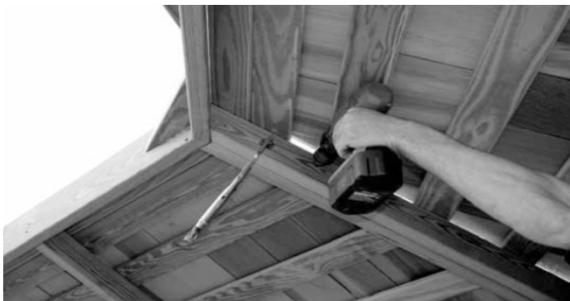
Tip: You can use several aides in aligning the rafters. A clamp is very handy in keeping the rafters aligned until they are secured to each other.
