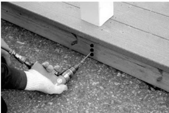
17. Now that both the top and bottom rails and top plate with fascia are installed you will want to go around the bottom of each post and secure the frame of the deck (rim board) to the posts. You will do this by screwing three 3 ½" screws into each outside facing post. This is very important because it will provide a lot of the stability for the Gazebo.
