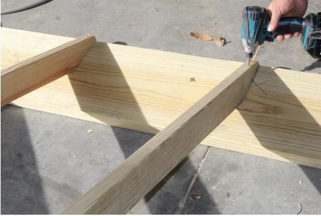
8. When they are fully secured to each other, attach the rafters to the top plate boards. Do this by aligning them over the pre-marked X's, and up against the inside edge of the fascia. Once in place attach the rafters to the top plate with 3 ½" screws, one through the top and one through the side of the rafter.
