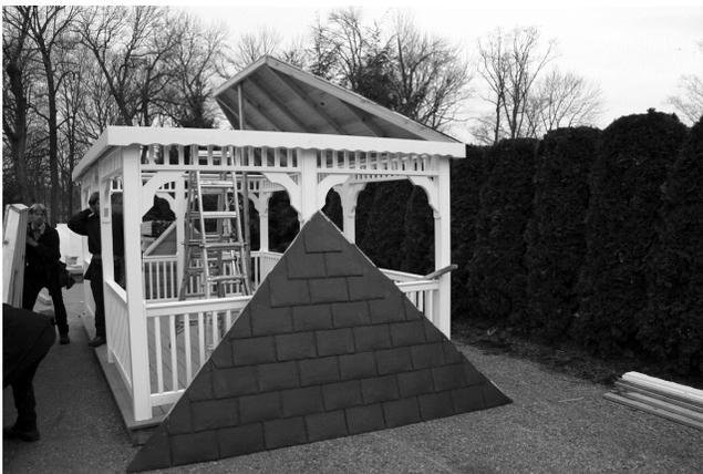
35. After you have the first section in place you can use a prop board to hold it into place while you get the second long side roofing section set into place. If you use a prop make sure that you place it toward the inside of the roof panel, so you do not have the chance of it see-sawing.
