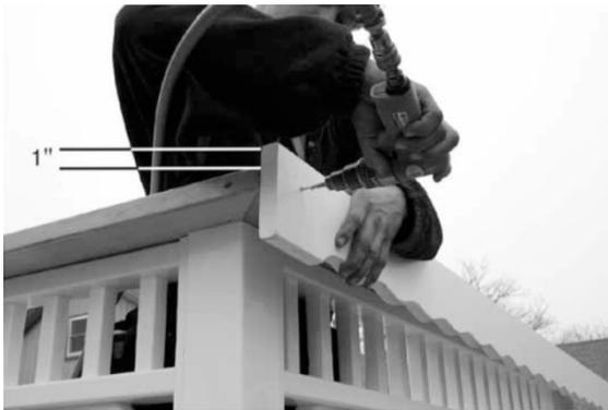
16. Now you can install the outside fascia. You will need to make sure that the fascia sets up 1" above the top plate. Once the fascia is in position you will want to screw it into the top plate with 2 ½" screws every 24". The screws should be 4" in from each end and 1 ½" to 1 ¾" from the top edge. Also the fascia may be a little long and will need to be cut to size.
