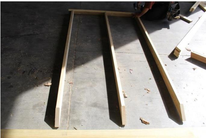
3. Next, find the center ridge rafters, these boards will be the same length and will have a matching angled cut on both ends like the picture shown. Make sure that the boards are laid out on the ground as shown.
