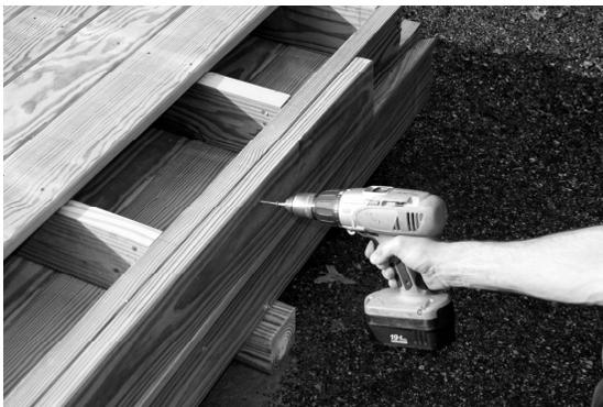
1. The first thing you will need to assemble is the floor of the structure. The floor is shipped to you in sections. Typically there are 2 floor sections but the floor may come in 4 floor sections for larger Gazebo's. You will need to first remove the boards attached to the end of the deck sections. (These will be used in Step #5)
