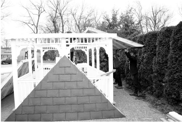
33. First raise a long side panel up onto the top plate. Slide this section up until the rafters in the roof drop into the top plate while resting against the inside of the fascia.
