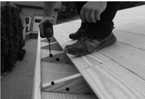
39. Use 2 1/2" screws to attach the rafters to the top plate. You will want to screw one screw into the top of each rafter and then also one into the side of each rafter.
