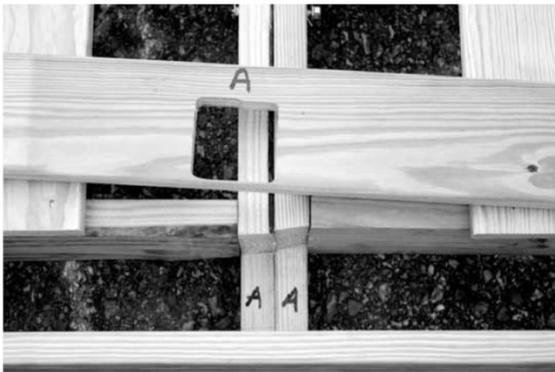
3. You will notice that there are letters on each joist that will join to another numbered or lettered section. Arrange each section with these numbers/letters as shown. Also the deck boards will have corresponding letters.
