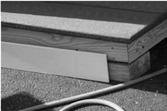
27. Gather all of the bottom fascia trim boards and place them along the bottom of the decking. Find the center of each deck side then, find the center of the corresponding floor trim board.
