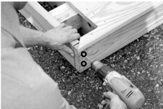
5. Next you will take the two decking ends that were removed earlier and you will want to screw them into place with 3  $\frac{1}{2}$ " screws. Screw the deck ends to the outside of the deck frame. After you have connected the exterior of the floor frame together you can now go back and tighten the bolts you set into place in the previous step.
