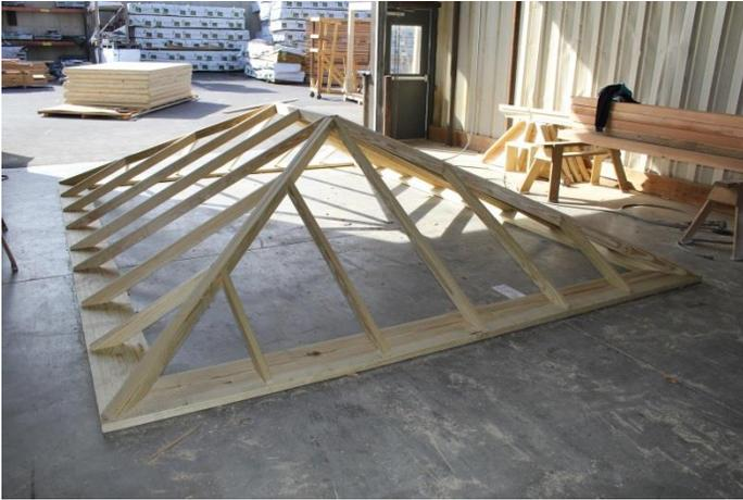
1. After you have installed the top plate and fascia boards, you are ready to start the installation of the stick built roof. To the left is an image of a 12' x 14' stick built Hip roof frame. This was built on the floor without the fascia.
